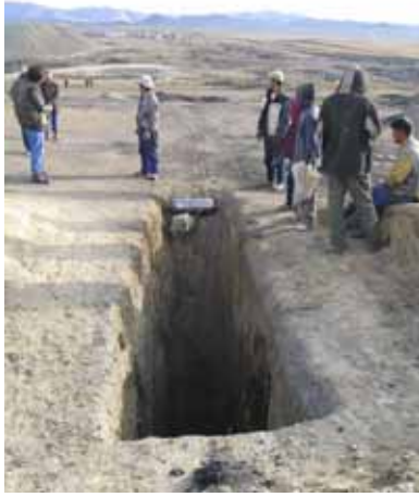
Figure 5. Inclined shaft for small-scale coal mining
